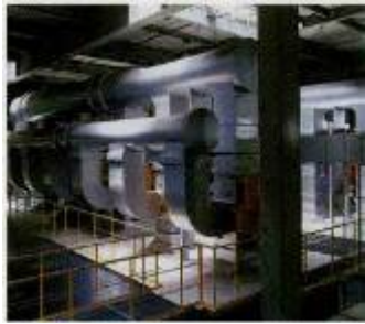
Flue gas treatment
